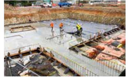
Above: The concrete foundations for the prefabricated walls at Resthaven Bellevue Heights.
