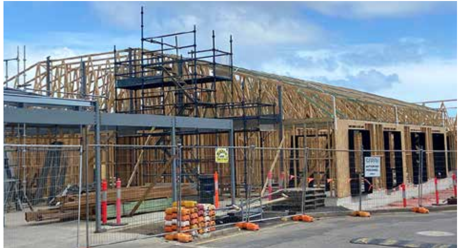
Above: Super structure under construction at Resthaven Bellevue Heights.
